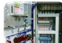
Panel Board Designing and Installation
